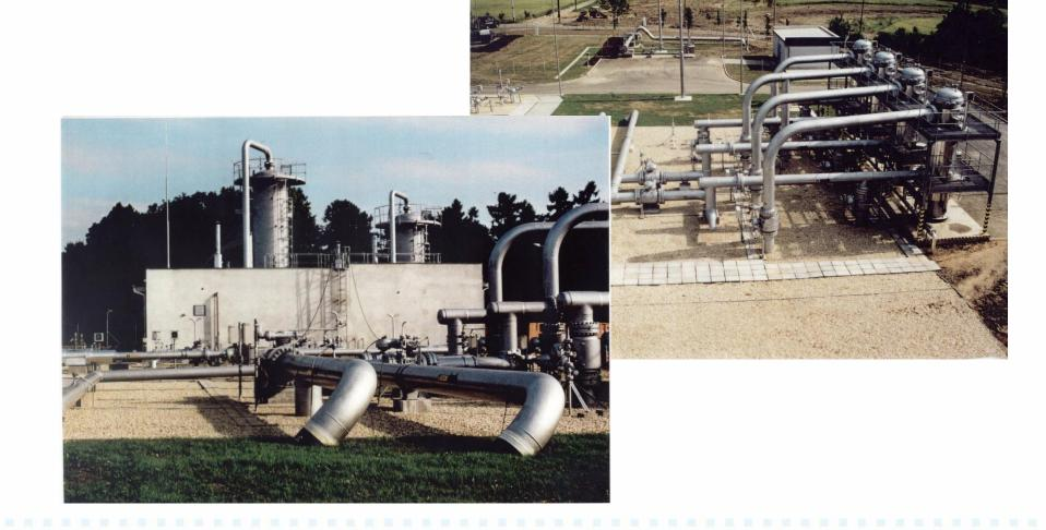
RWE Gas Storage, UGS Dolní Dunajovice, Filterseparators for Natural Gas
