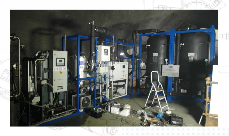
» 2018 – Radon Removal System, China Shanghai Jiao Tong University, located at Jin Ping Underground Laboratory, China
